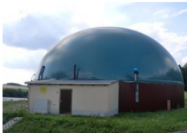
75 kW Gülle-Biogasanlage in Clausnitz
